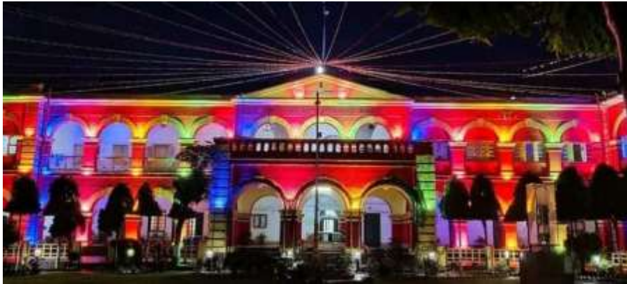
DGMS HEAD OFFICE, DHANBAD
